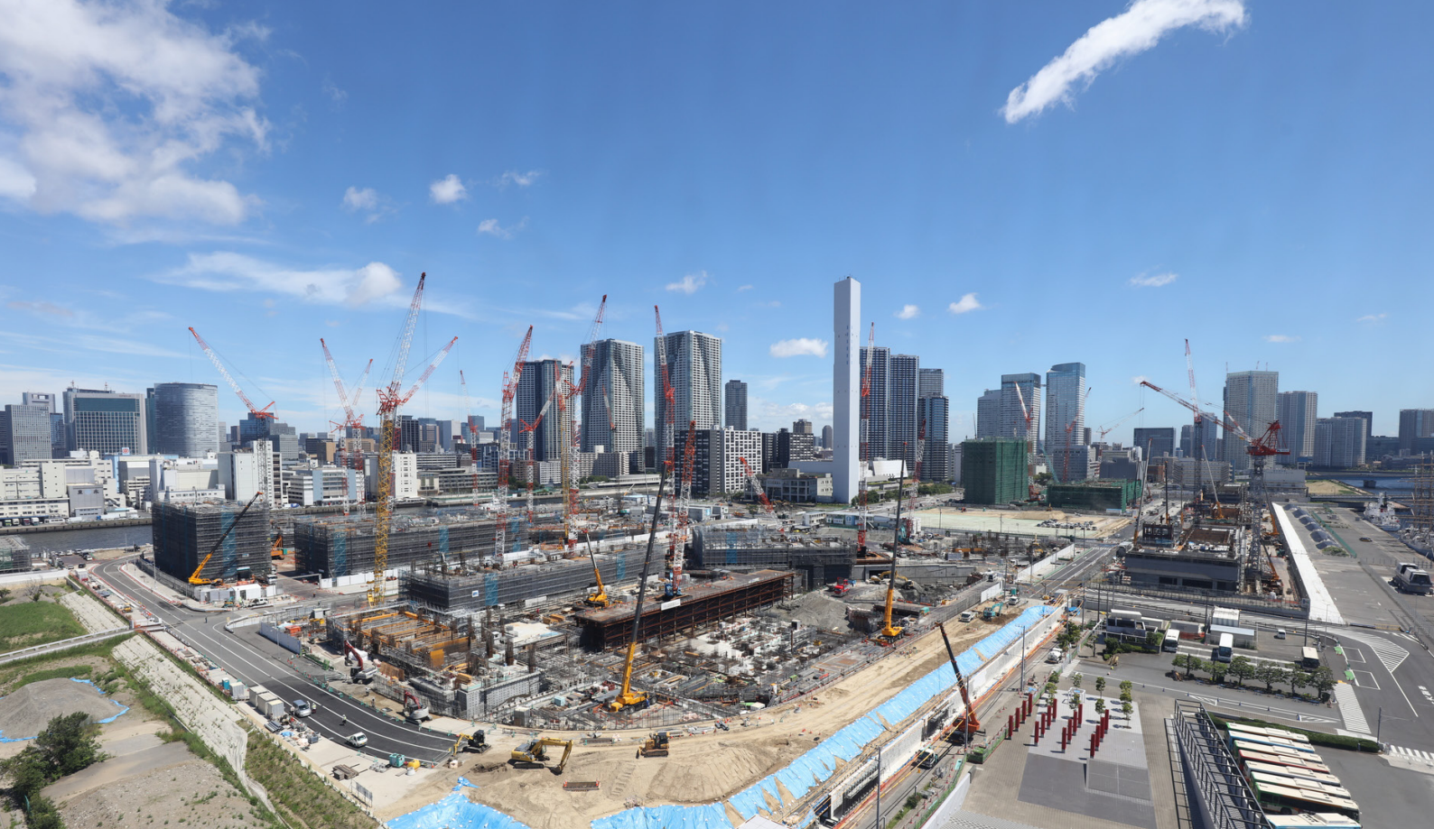
Olympic Village under construction as of June 2018
